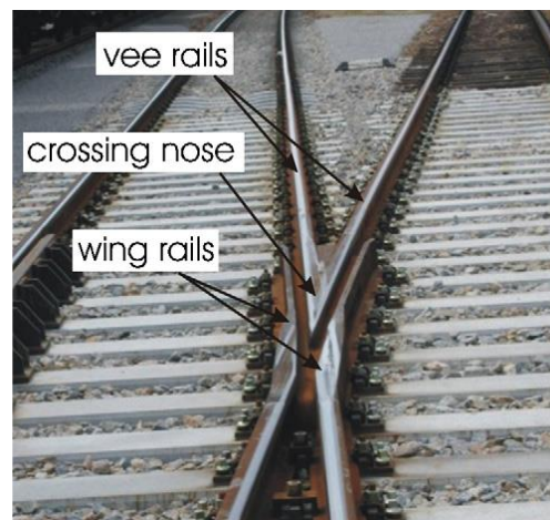
Figure 4. Typical casted manganese crossing [25]
